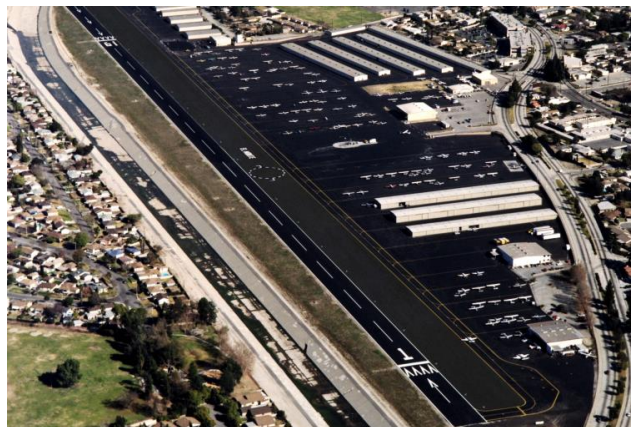
Figure 6. El Monte airport in Los Angeles county treated with REAS in 1994
